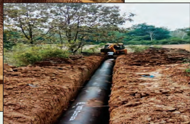
Laying of Pipelines & other structural works at Baripada block by RWSS Baripada division.
