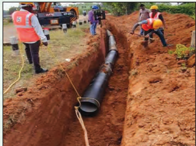
Laying of D.I K-7 pipeline in Jagannath Sahi of Vyasaganar ULB.
