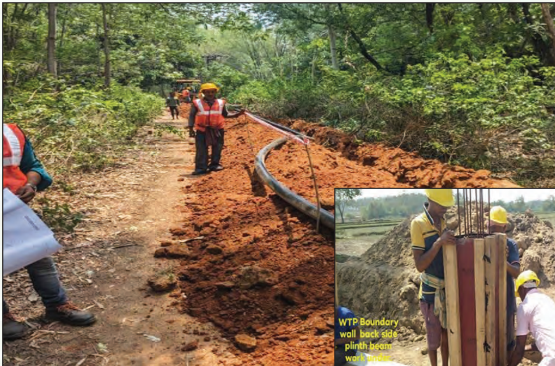
Construction work in WTP & Laying of Pipelines at Raruan & Sukruli block by RWSS Rairangpur division.
